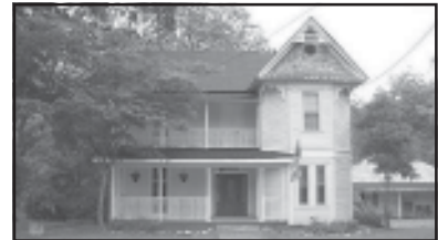
OXFORD - NEWTON COUNTY - Beautiful 5 bedroom, 3 bath Victorian home, just waiting for a family. Nice hardwood floors, ceramic tile in kitchen & baths, tray ceiling in dining room. $199,000. GAMLs #2673179
