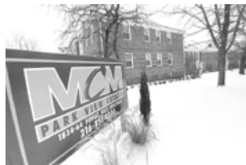
Some areas south of Euclid Avenue are well-kept, like landlord Ted Lichko's apartment complex near Forest Hill Park.
