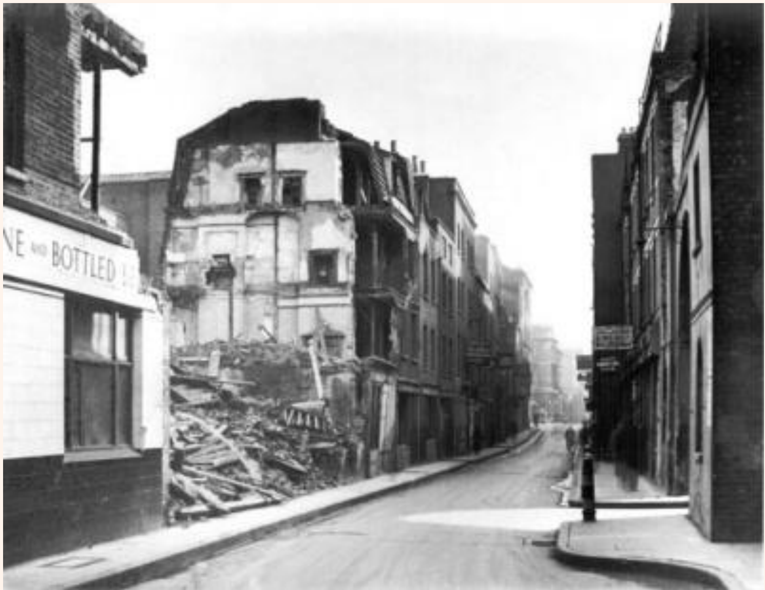
White's Row looking east, showing bomb damage, 1943.
