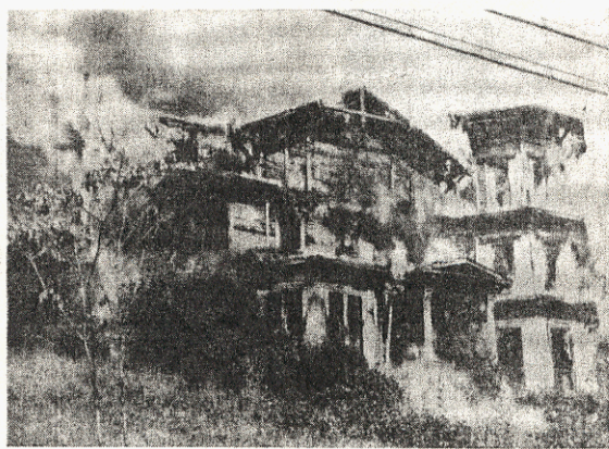
Once proud mansion of Wallace family, old Assumption Convent, facing North Main Street, scorched by parish in 1907 from Thomas and Ellen B. Wallace, ended its career in flames Wednesday afternoon. Building was over 70 years old.
