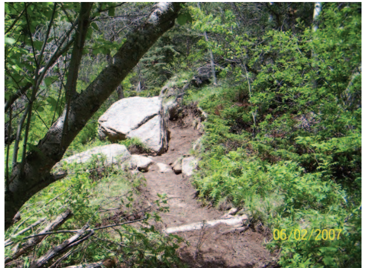
One of our many successful trail repairs
