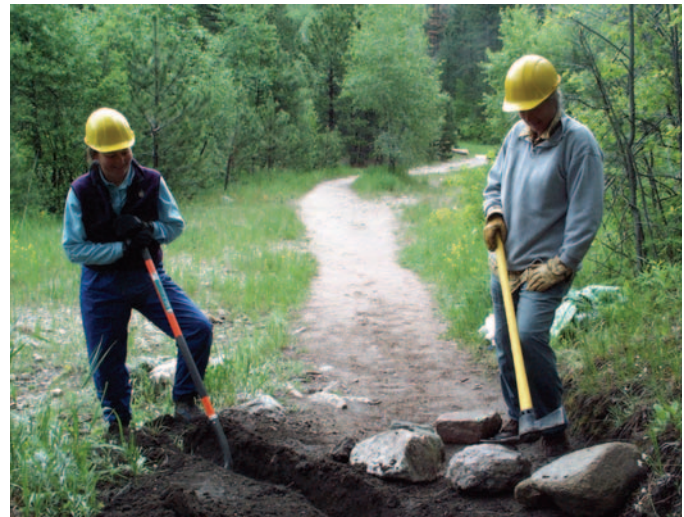
The trench and rocks for the water bar
