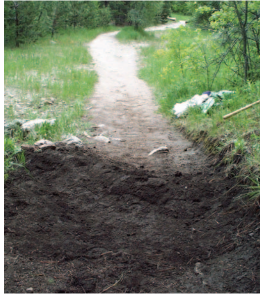
After we put in the water bar: We have since seen that this water bar continues to protect the trail from erosion due to water running down the tread.
