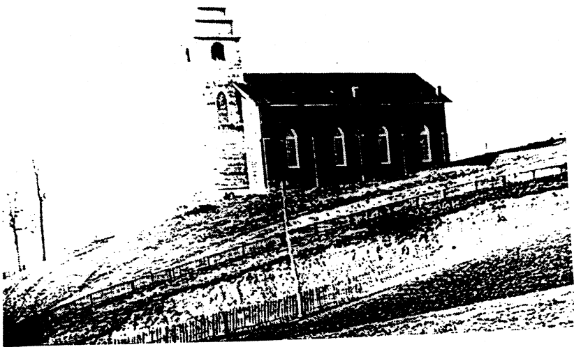
CHURCH WITH HIGH STEEPLE
