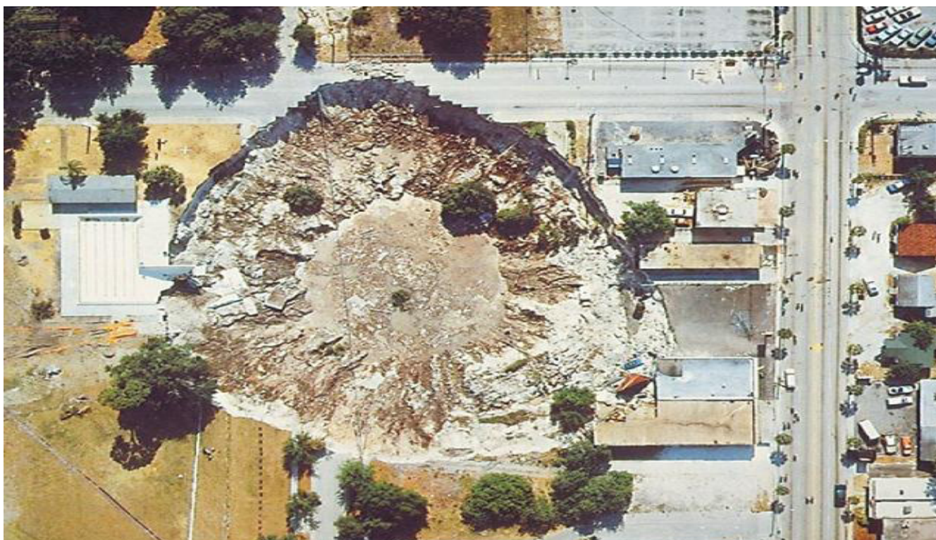
This sinkhole developed in Winter Park, Florida, in 1981.
