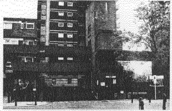
Shearsmith House (before)
