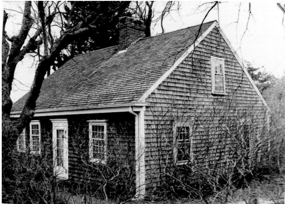
Home of John Ellis (d 1677), Sandwich, built 1647, still standing
